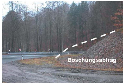
Figure 11: Removal of sight barriers in curves 11
