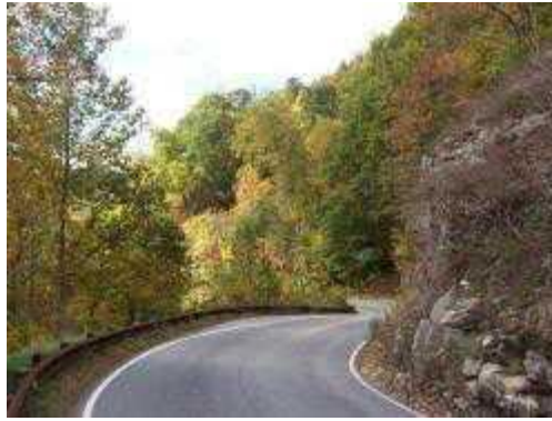
Figure 14: Dangerous obstacles in bends 13
