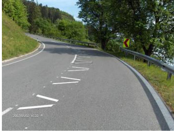
Figure 10: Floor markings for enhanced lane separation in curves 10
